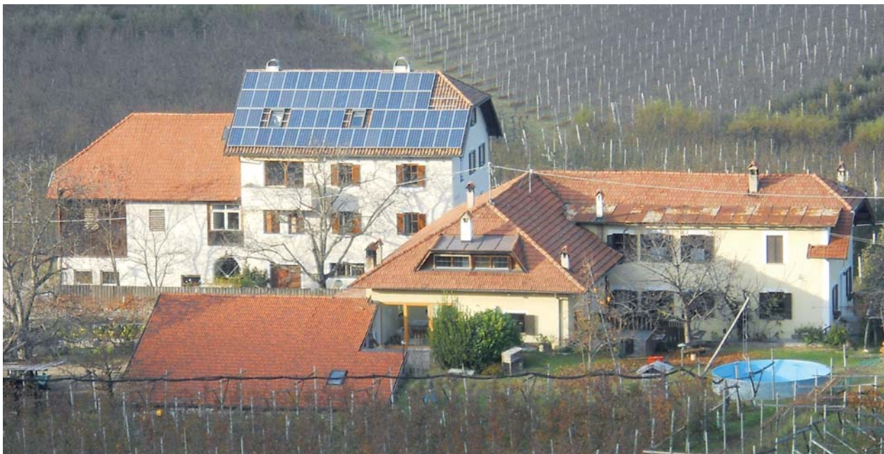
Photovoltaikanlage in Eppan
